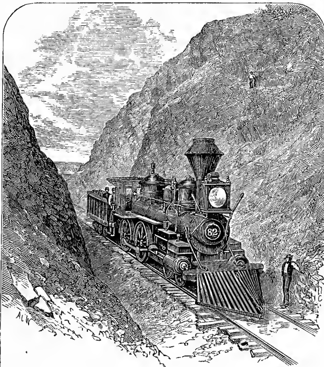
ROCK CUT, NEAR ASPEN.
