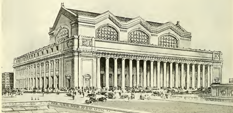
NEW UNION STATION, CHICAGO (Under Construction)
