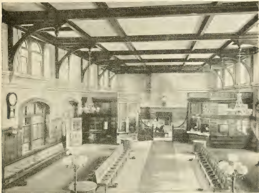
FIG. 633. PERSPECTIVE OF INTERIOR OF WAITING-ROOM.
