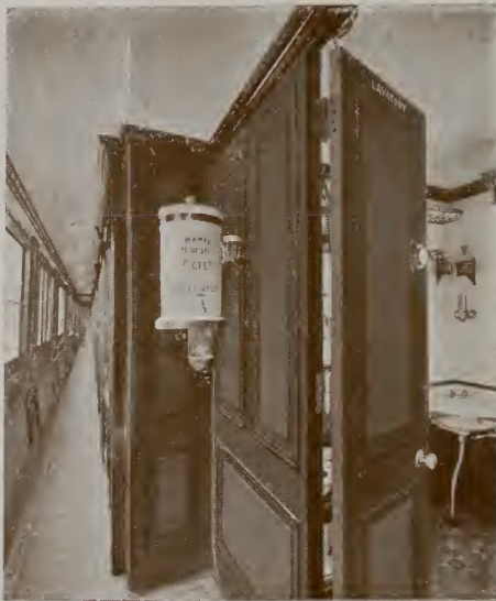
CORRIDOR AND LAVATORY.
