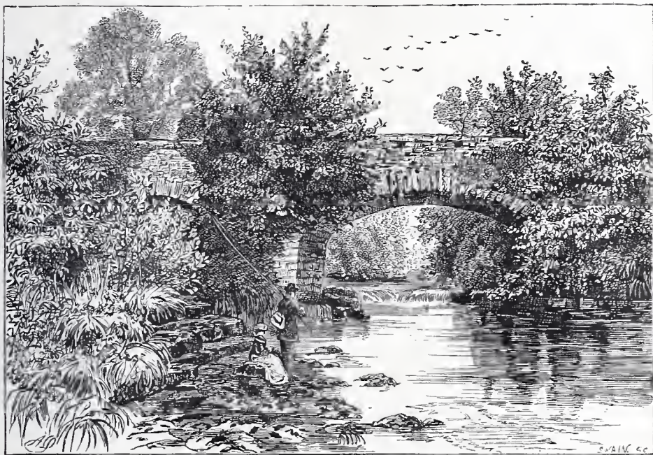
HAWES BRIDGE, KENDAL.
