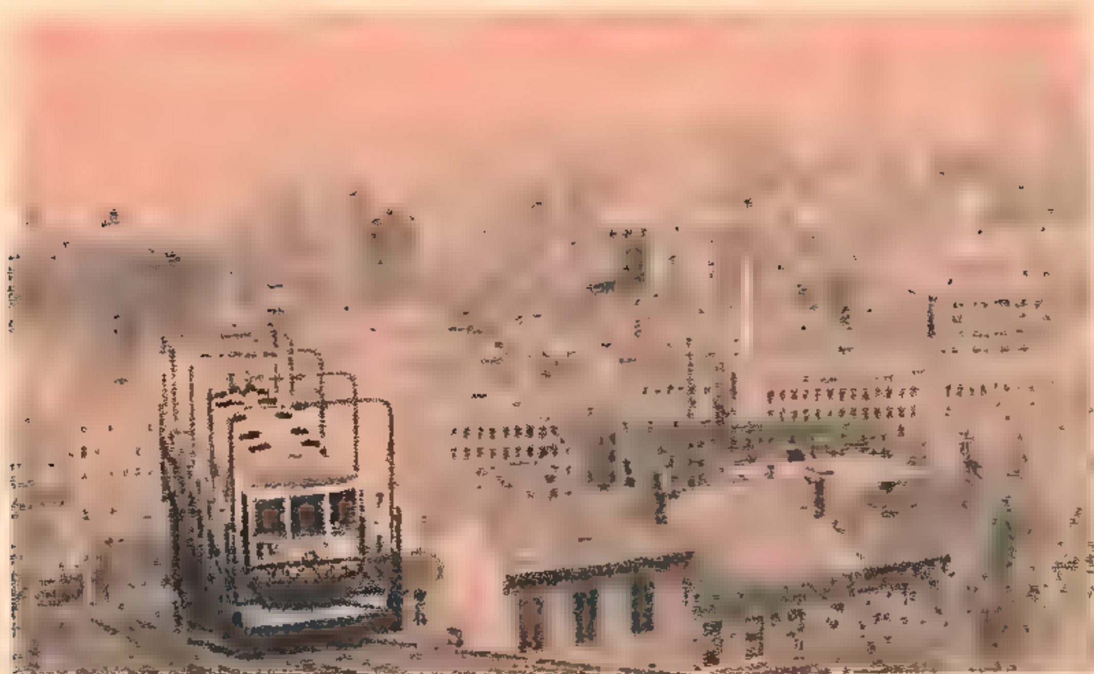
Street cars carrying tourists are the principal users of this old plane railway in Cincinnati, Ohio. The cable lifts carry the cars up a 980-foot incline featuring a grade of 28.9%.
