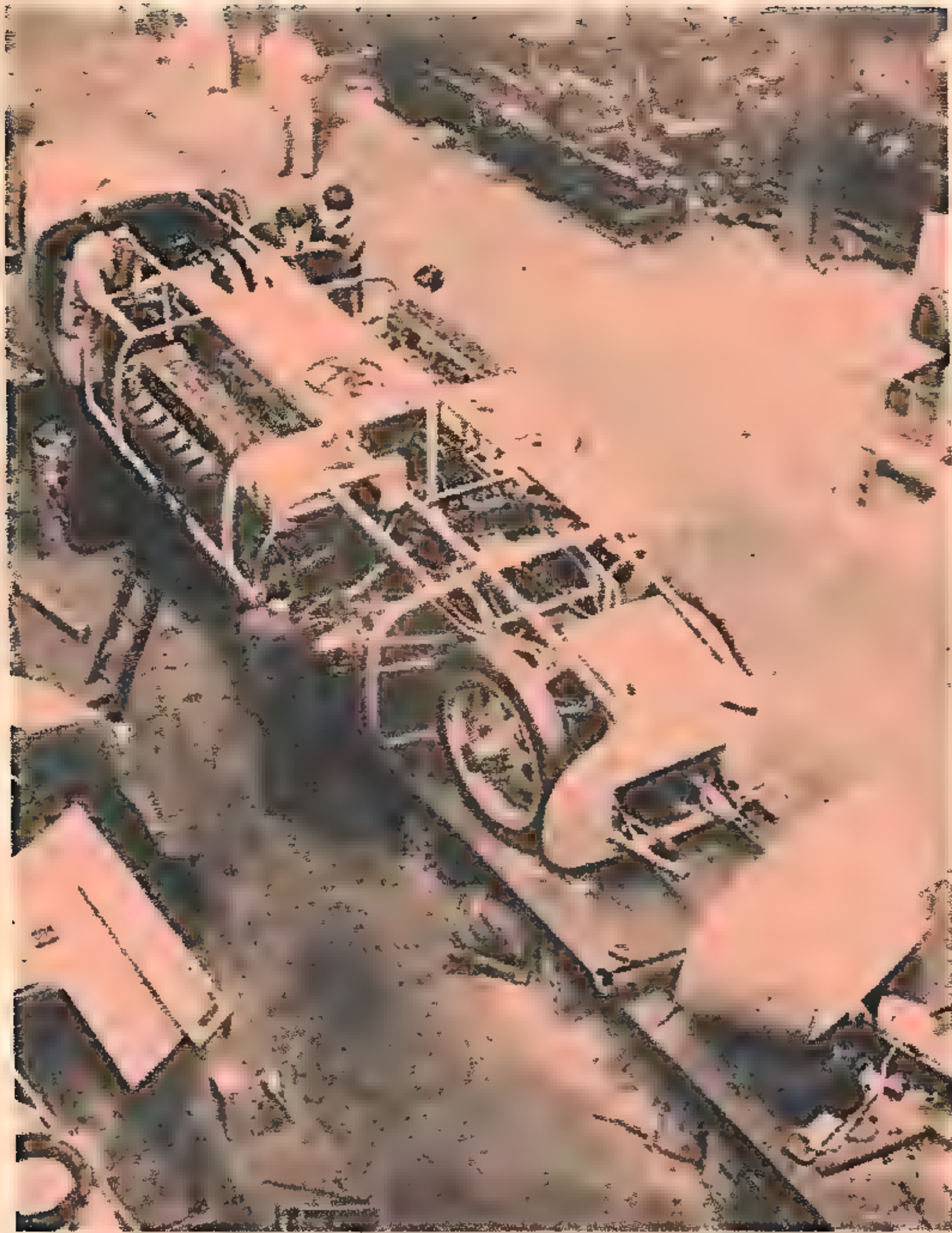
This 36-foot racing car is being built for Captain George Eyston, of England, who hopes to attain a 400-m.p.h. speed with it. When completed, the racer will have eight wheels.
