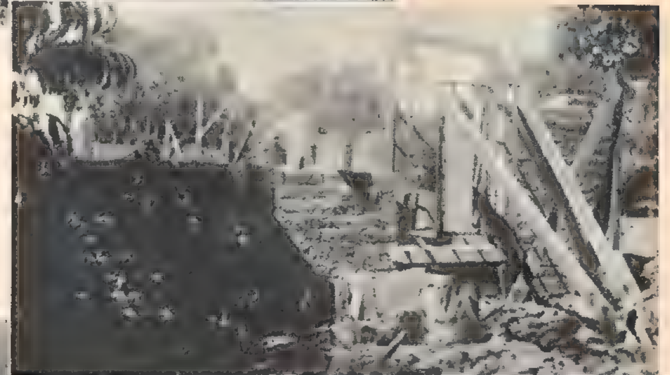
The roof rafters, of native timber, are supported at the ridge by a log extending through each gable end wall, as shown in above photo. Right—Setting in the window frames. Below—When completed, the outside of the novel house is whitewashed to create a real Spanish appearance.
