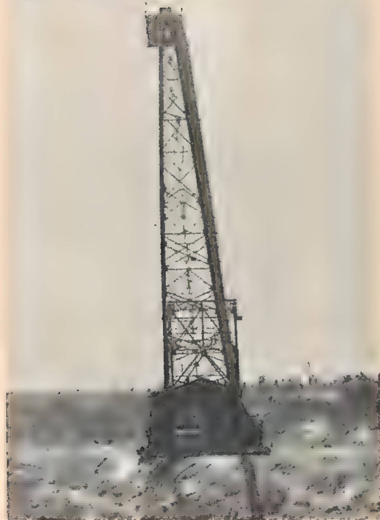
Elevated skyward, the boom of this huge dragline looks like an oil derrick. In operation, the boom enables the dragline bucket to go into action at any point within the boom's radius.
