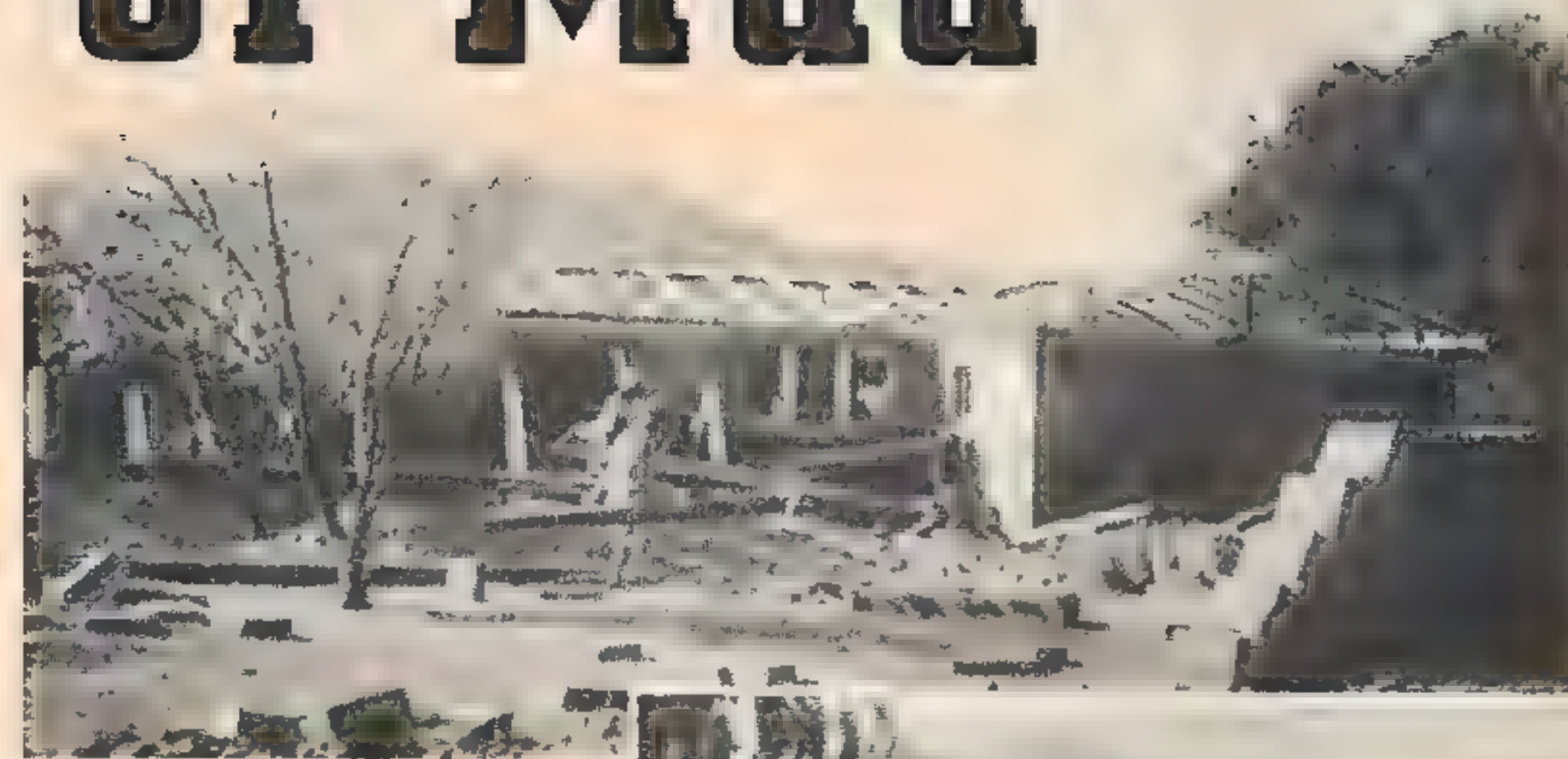
The roof rafters, of native timber, are supported at the ridge by a log extending through each gable end wall, as shown in above photo. Right—Setting in the window frames. Below—When completed, the outside of the novel house is whitewashed to create a real Spanish appearance.
