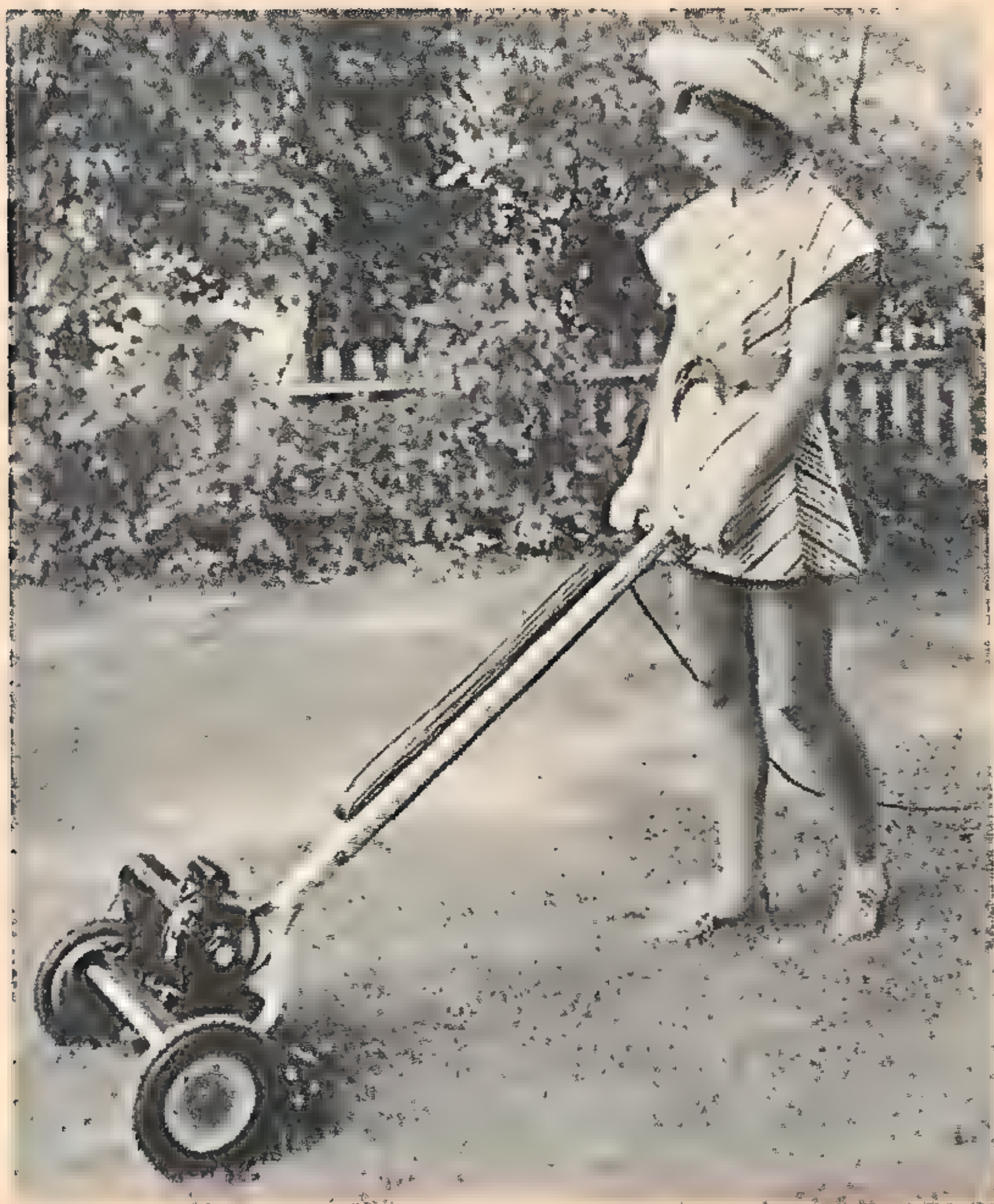
Unusually quiet in operation, this rubber-tired electric lawn mower need only be guided over a lawn, since it is motivated by a compact one-quarter horsepower geared motor.
