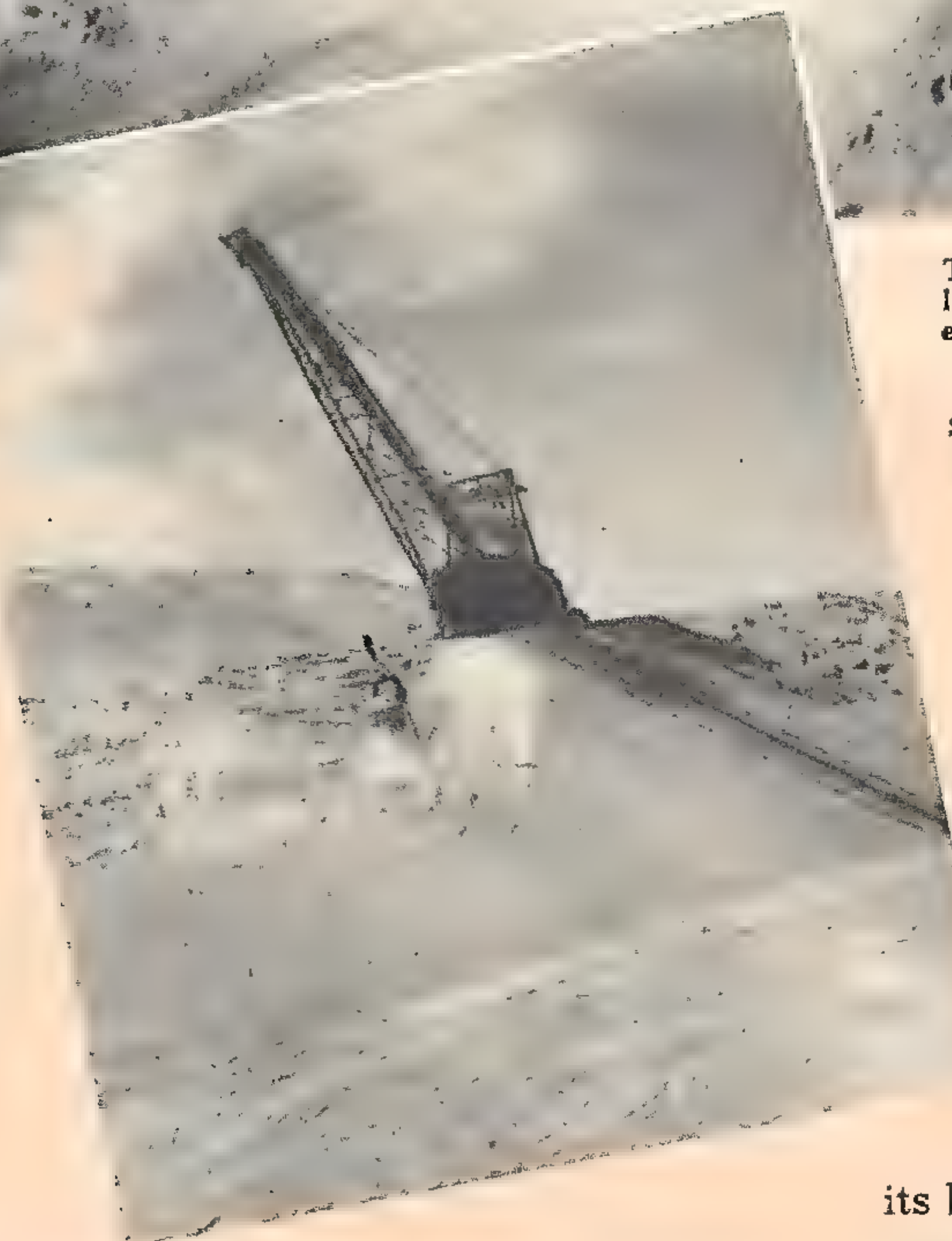
This dragline scoops up enough dirt in one "bite" to fill a waiting truck to overflowing. Note men at work in pit.
