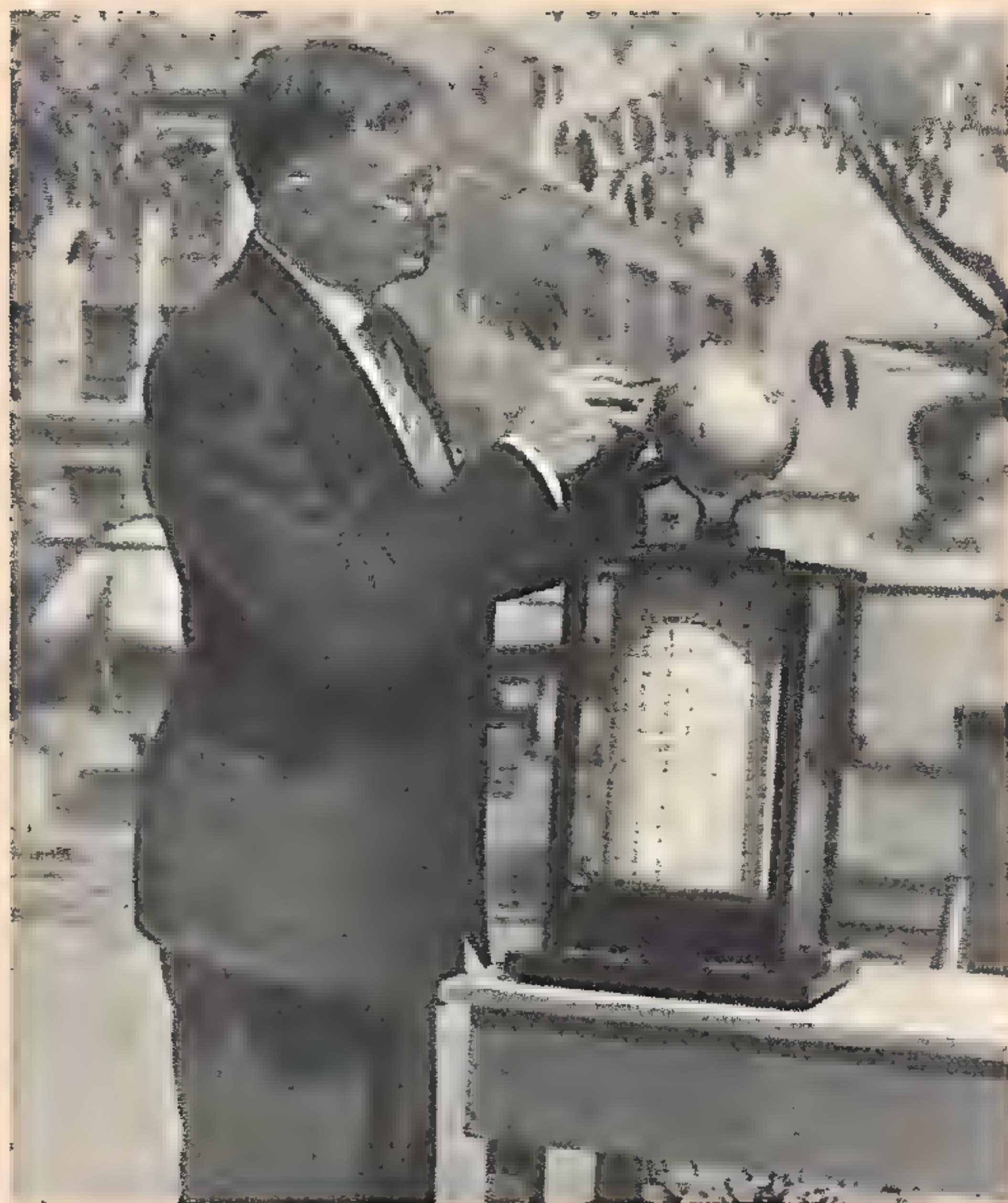
Designed primarily for short-wave enthusiasts and airport use, this universal electric clock simultaneously indicates the correct time at 16 large cities scattered over the globe.
