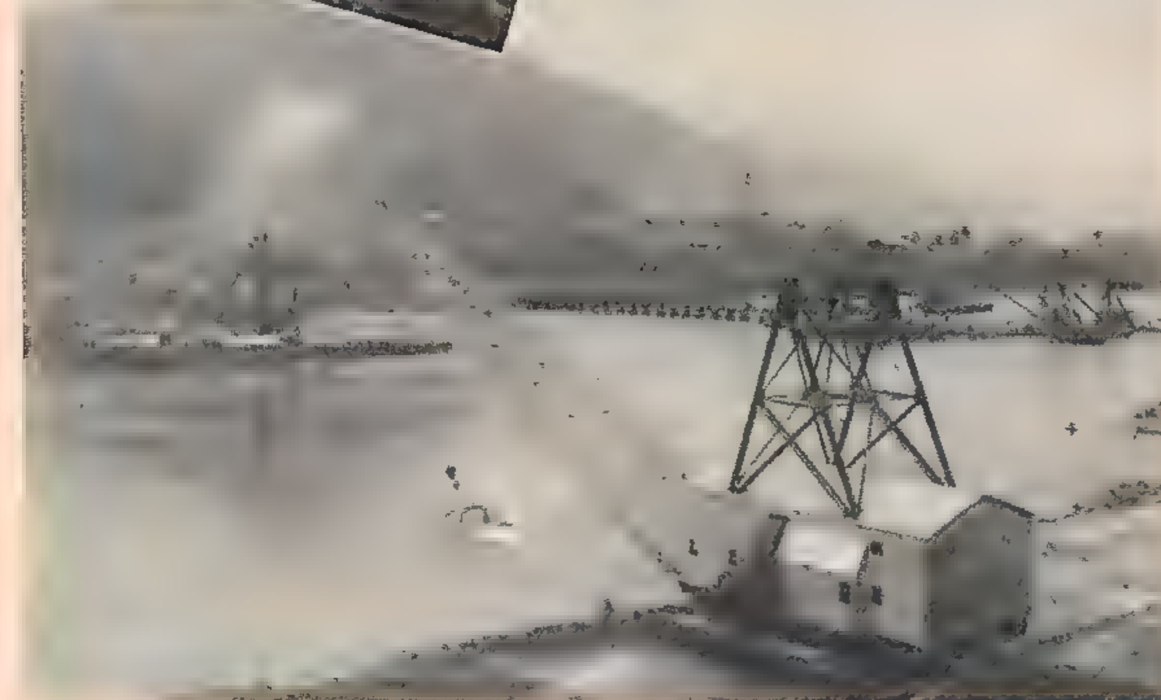
One of the biggest draglines in the world (above) at work in an Iowa coal mine. The machine reaches down into the cut, strips overburden away, gouges out a load, and swings it back out of the way. One bucket load represents work of hundreds of men.
