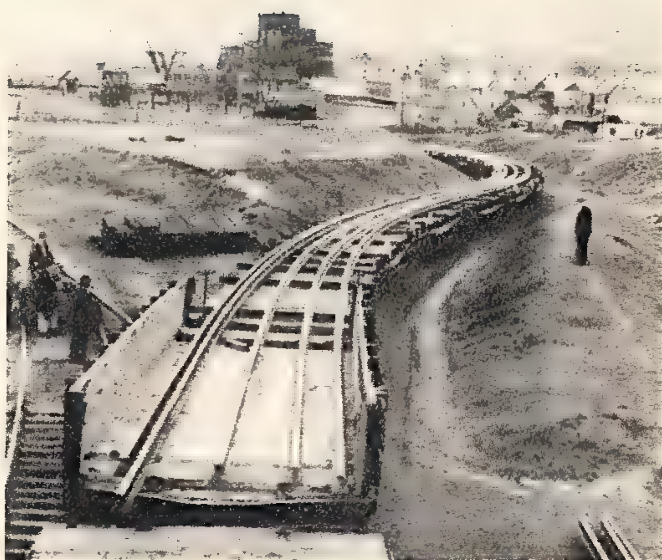
Flexible enough to bend around a 15-degree curve without being fastened to the flat cars, a mile-long continuous stretch of welded track is carried to a Pennsylvania test site.
