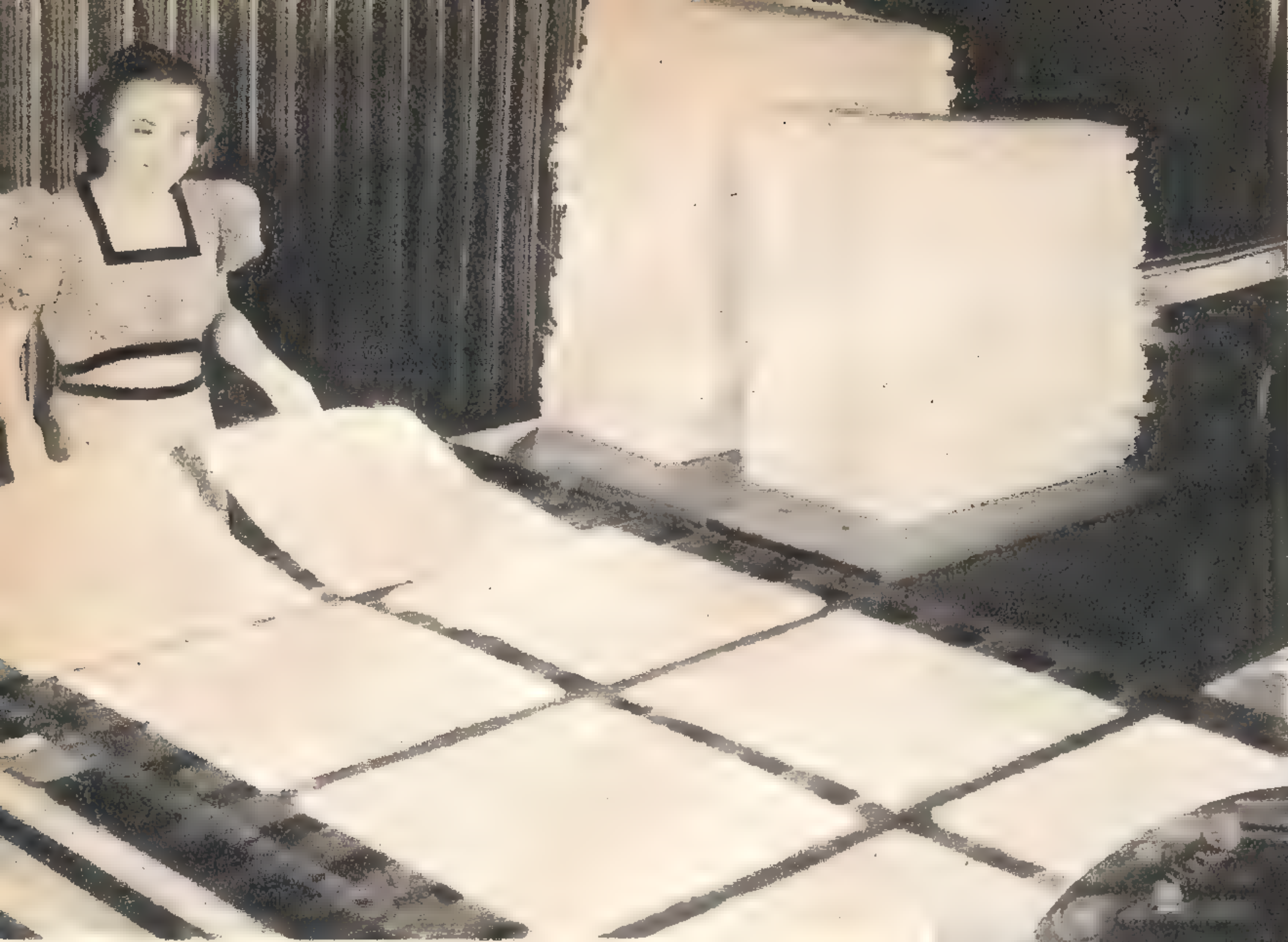
Left: These thin mats, composed of thousands of strands of Fiberglas, are used as air filters for warm air furnaces, and industrial machines operating in dusty atmospheres. This is one of the many applications of "glass cloth."
