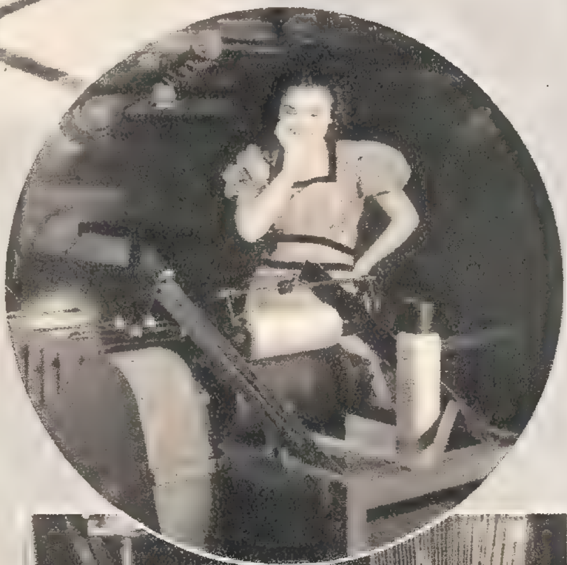
Below: Fascinating to watch is this "staple process" of forming glass threads. The molten glass is blown down past the drying flame at the edge of the picture, and forms almost out of thin air as fine white threads, which are taken up on the spools.
