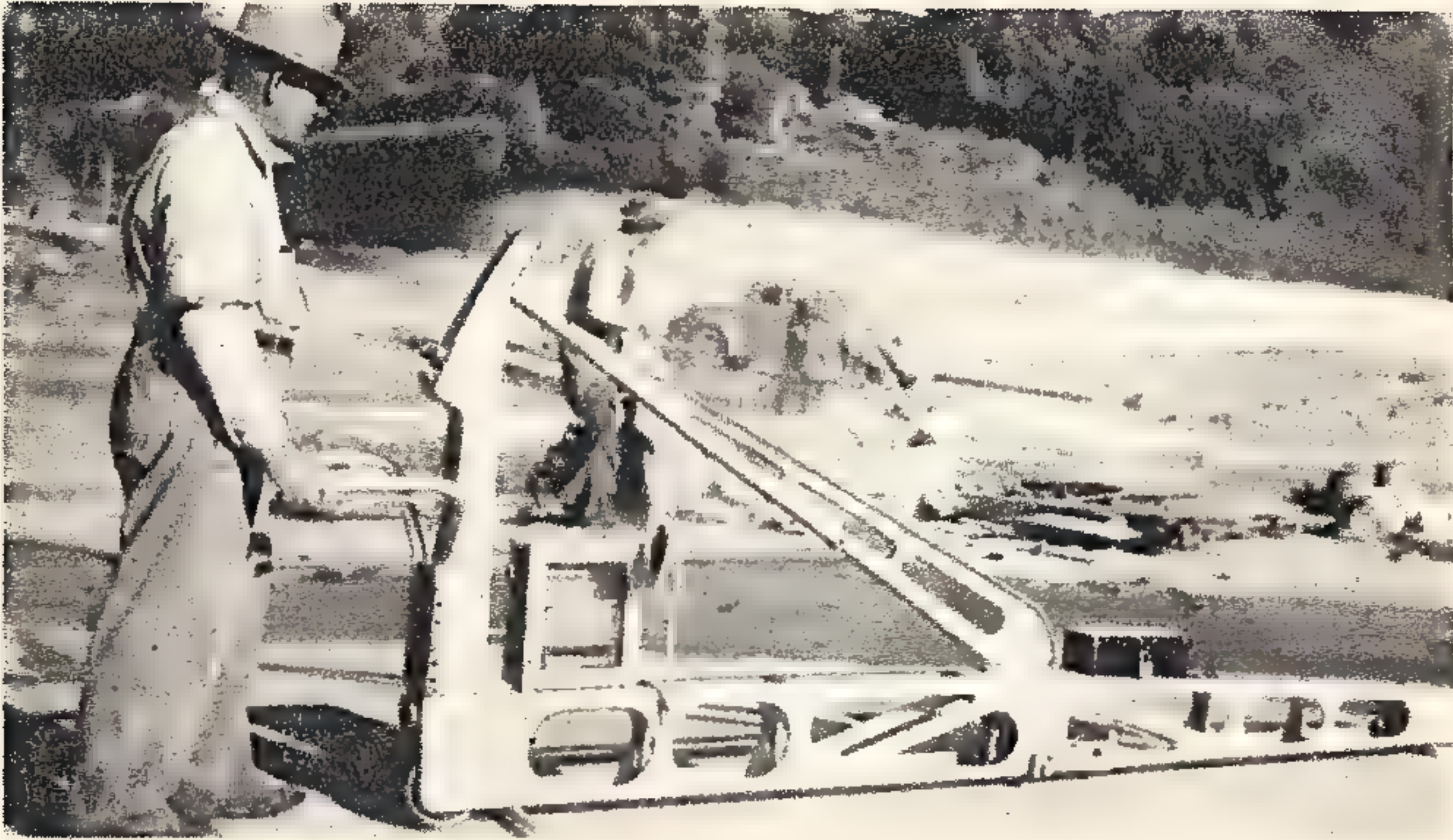
Deviations in highway pavement as small as 1/100th of an inch are readily detected and magnified by this "Planeometer" device, which is used by Oregon State Highway Commission.
