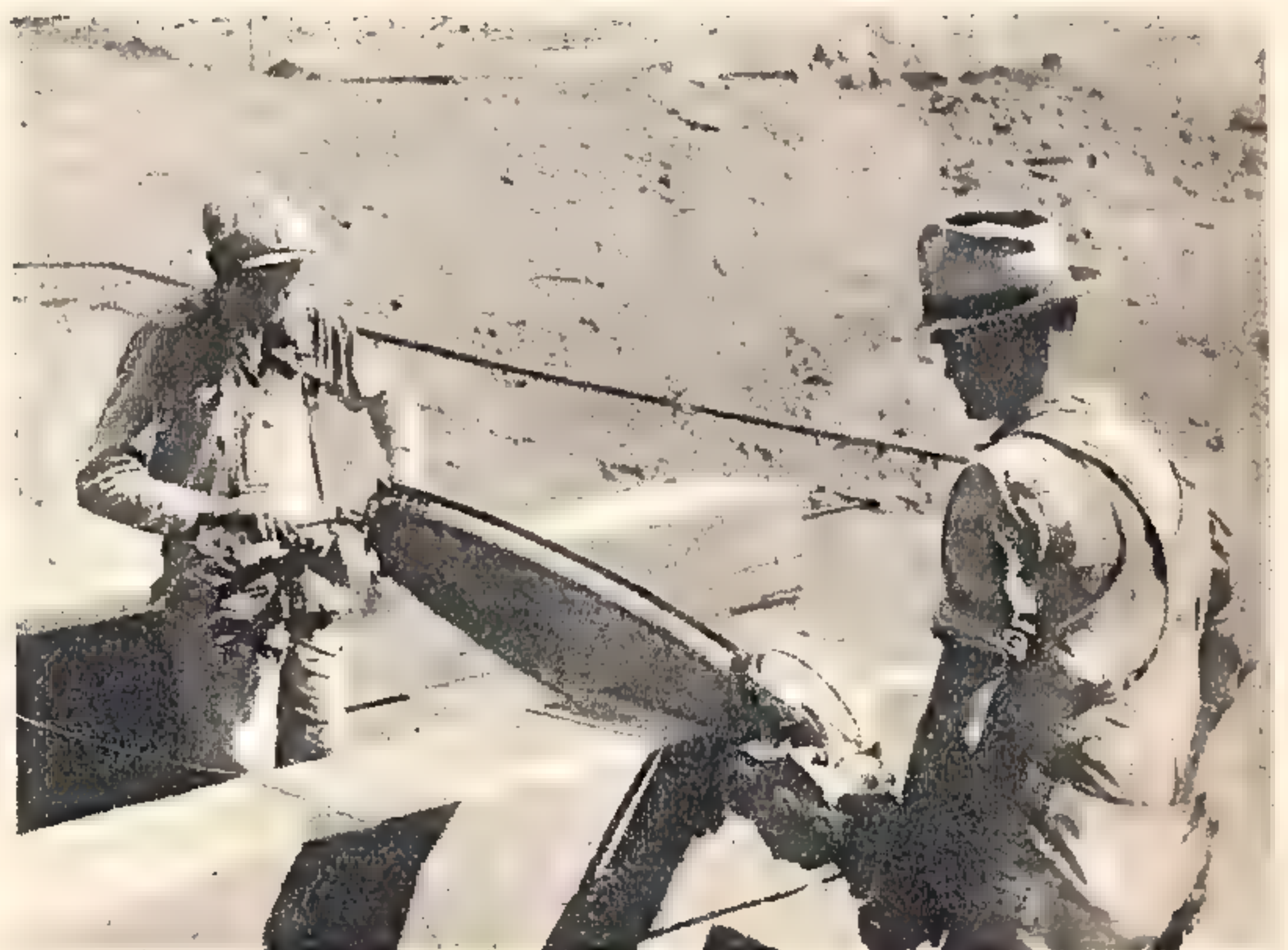
These workers are using a novel saw featuring a blade that stands still! The cutting teeth run around the blade on an endless chain, which is powered by a compressed air motor.
