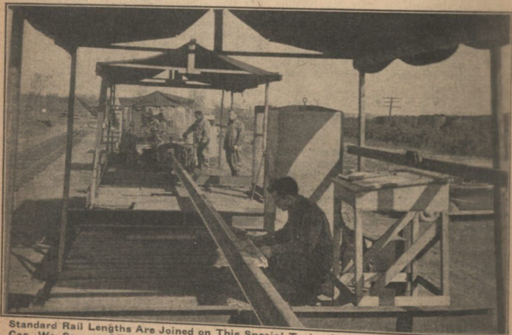
Back in 1933, the Delaware & Hudson Laid 12,075 Feet of Continuous Rail at Albany, N. Y. Since Then More Than Ninety-five Millions Tons of Equipment Have Rumbled Over This Test Section, Convincing the Road That It Was Well Worth the Extra Cost of Installation. Eleven Other Stretches Are Now in Service. The Longest Single Butt-Welded Rail Has a Length of 7,018 Feet
