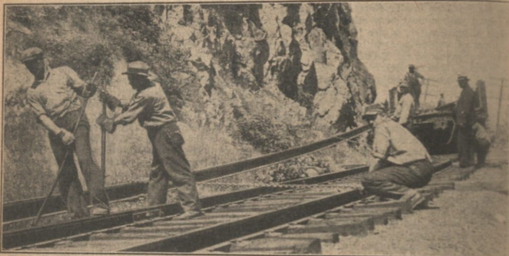
Back in 1933, the Delaware & Hudson Laid 12,075 Feet of Continuous Rail at Albany, N. Y. Since Then More Than Ninety-five Millions Tons of Equipment Have Rumbled Over This Test Section, Convincing the Road That It Was Well Worth the Extra Cost of Installation. Eleven Other Stretches Are Now in Service. The Longest Single Butt-Welded Rail Has a Length of 7,018 Feet
