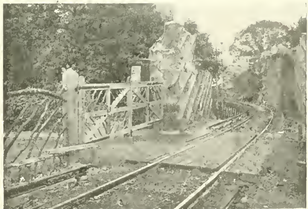
Level Crossing at Upper End of Trestle Bridge, Showing Jumper Cable Connections.
