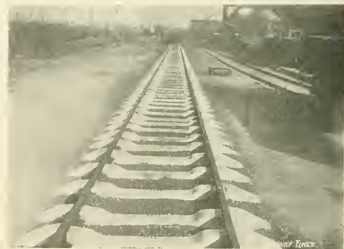
Concrete Sleepers under Test on the Pennsylvania Railroad.
