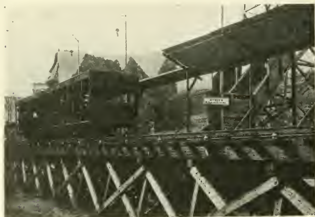
Train on Trestle near "New Zealand Station."
