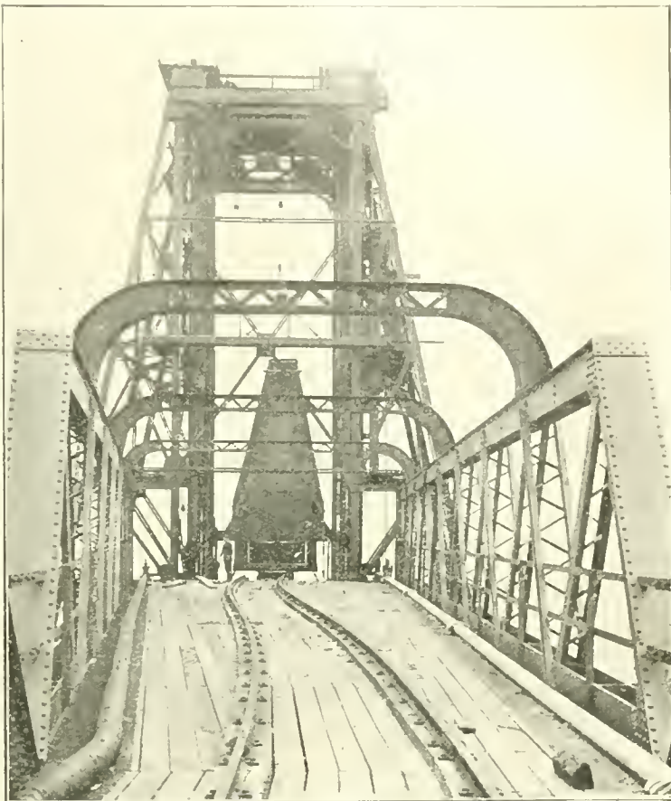
West Jetty Coal Hoist, Immingham Docks—Capable of Shipping Coal at the Rate of 700 Tons per Hour.
