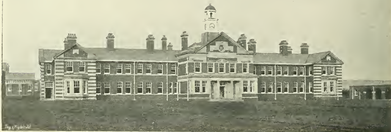
The "Webb" Orphanage at Crewe.
