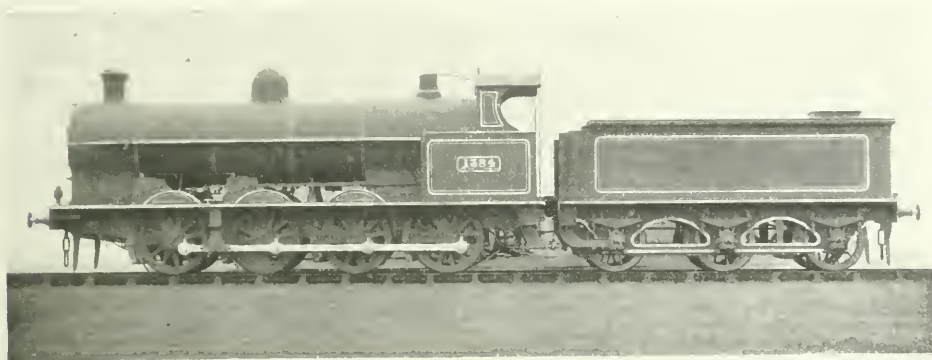
Eight-coupled Superheated Goods Engine—London and North Western Railway.
