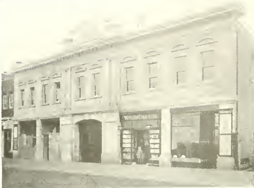
Facade of Ealing Station.
