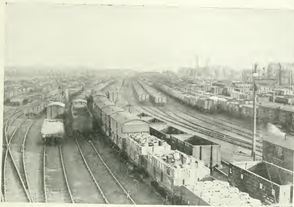
General View of Sidings at Willesden Junction. All Work Suspended.
