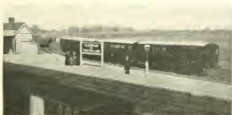
Light Railway Train at Elsenham Station
