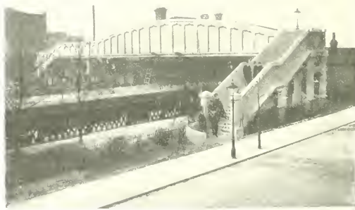
Ferro Concrete Foot-bridge, Kew Gardens Station London & South Western Railway.
