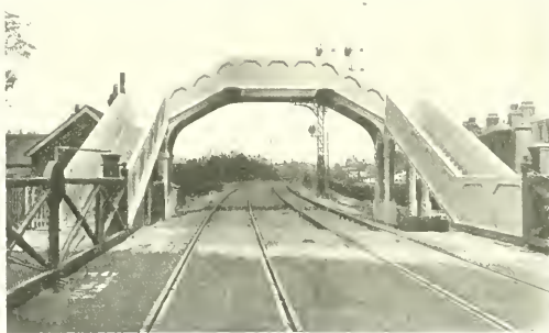
Ferro Concrete Foot-bridge Over Line
