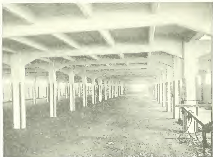
A Floor in the Warehouse Lambeth Depot
