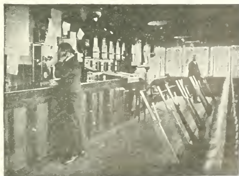
Way Station Selector Set in Signal Cabin
