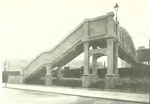
Ferro Concrete Foot-bridge, Kew Gardens Station London & South Western Railway.
