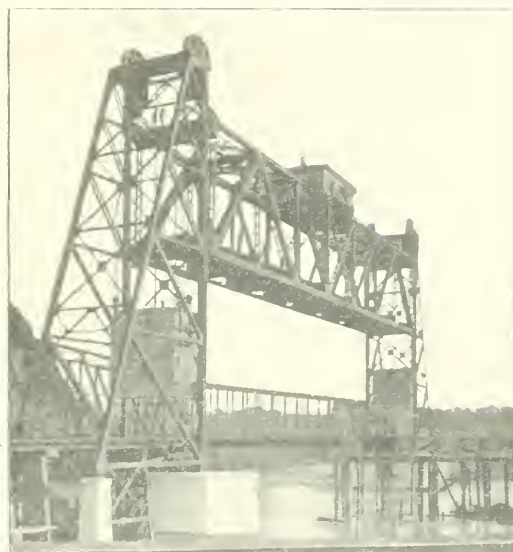
St. Paul Railway Bridge-Span Subject for Investigation
