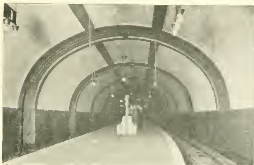
Hauptbahnhof Underground Station with Island Platform
