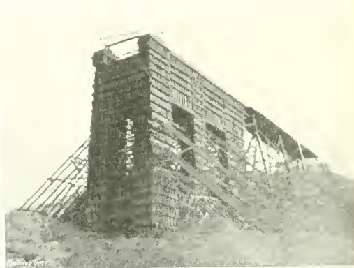
Fig. 3.—Wooden Forms about Abutment ready for concreting.
