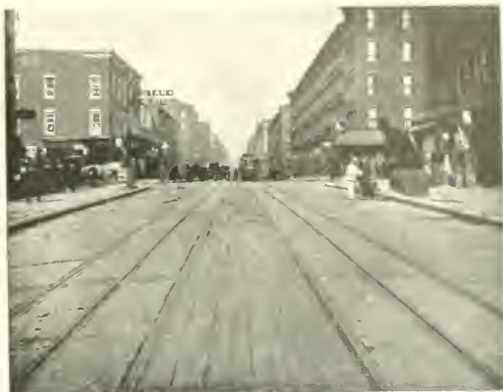
Surface of Lexington Avenue during Construction
