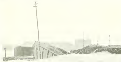
Franklin Bridge at the moment it fell
