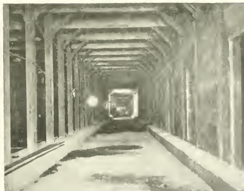
Section of Partially Completed Subway directly beneath above scene
