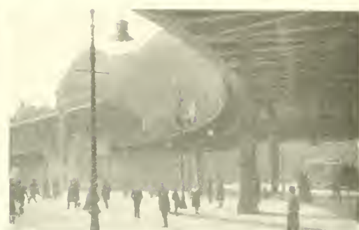
Overhead Structure on Curve and Rodingsmarkt Station
