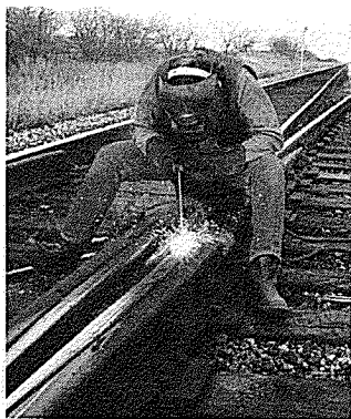
Left: Division Welder Buddy Andrews works on "frog" at entrance to the new 11,000-foot siding at Caldwell, Texas. Above: Installing an automatic switch machine at Caldwell under supervision of Foreman James Josey (white hat) are (left to right) signal gang members Wayne Bennett, Rickey Colonga and Dennis Ganston (at crane controls).
