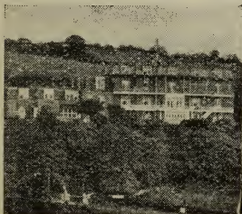
View of Hotel taken from Harbour.
