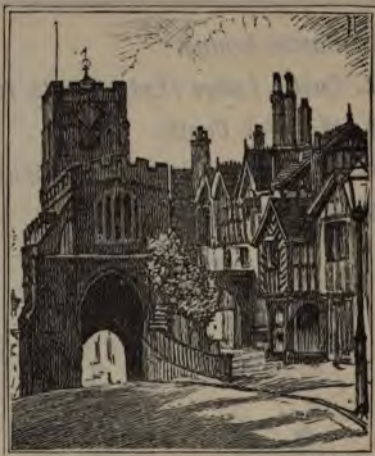
GATEWAY OF LEICESTER HOSPITAL, WARWICK.
