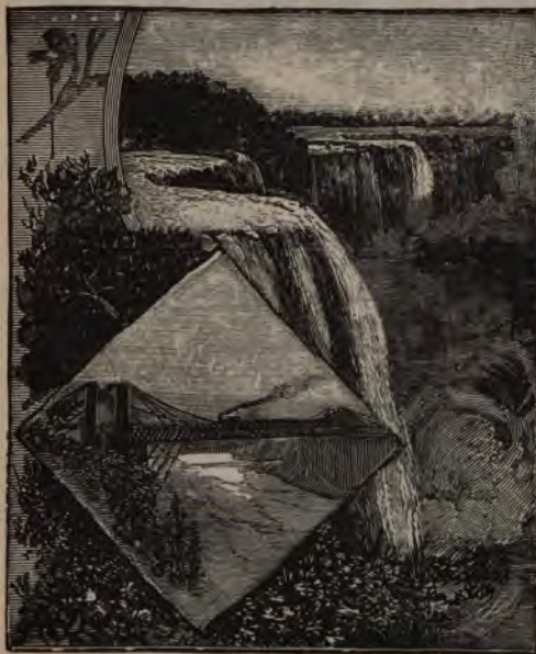
SUSPENSION BRIDGE AND NIAGARA FALLS.
