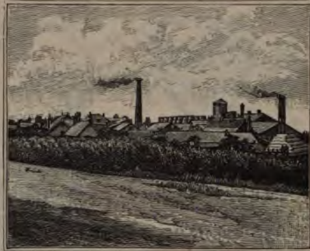
THE RUGBY PORTLAND CEMENT WORKS, RUGBY.
