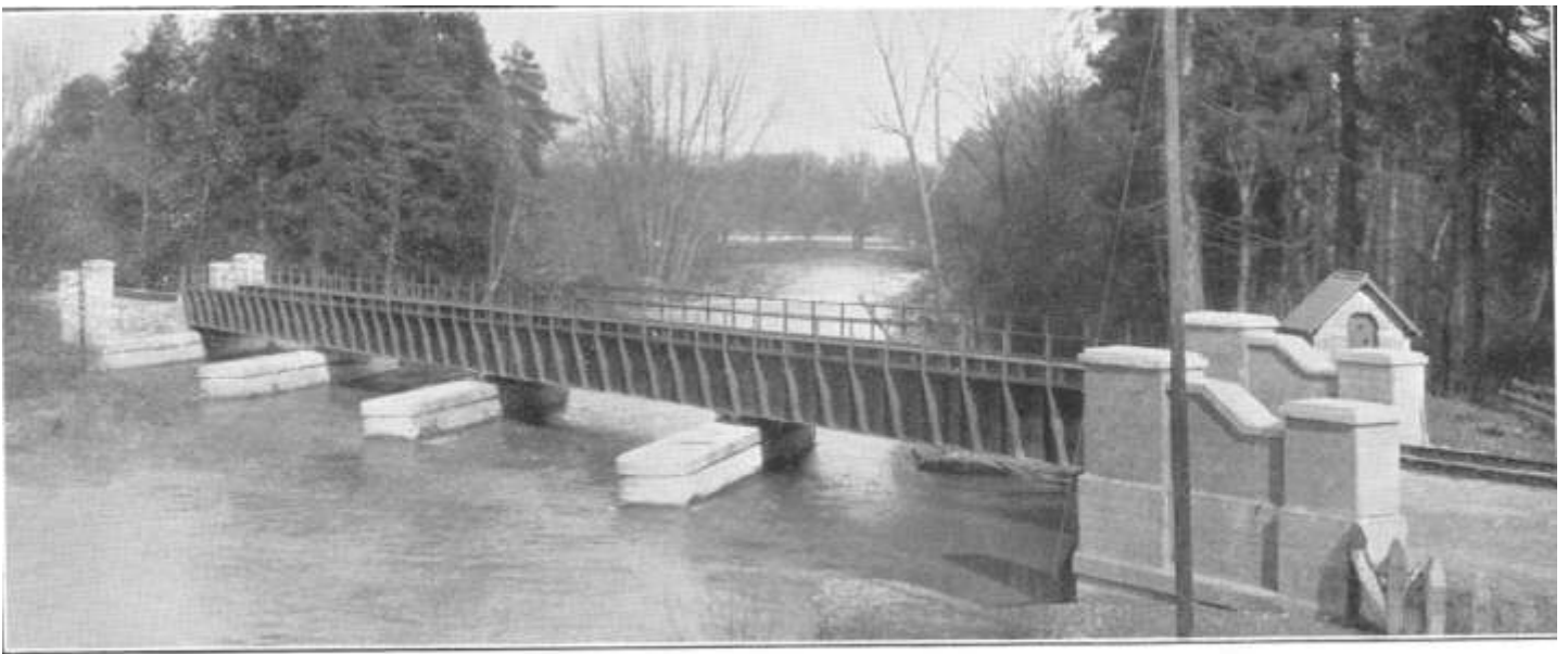
KILKEWYDD BRIDGE, near Welshpool, as recently re-built.
